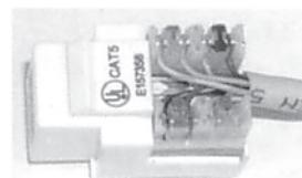
Hold tightly with cable jacket by cable tie to avoid the cable knock off or pulling away, then complete the installation.
