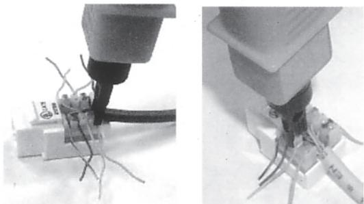
Use the impact tool to crimp and connect the wires.
